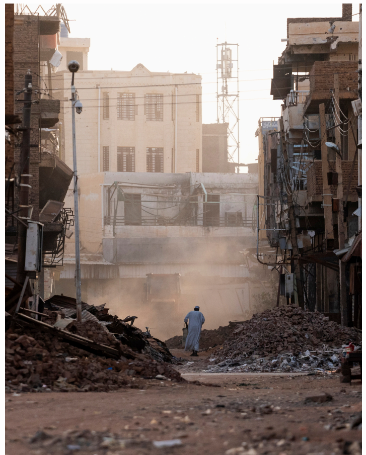
People pass through a destroyed section of Omdurman, Sudan, on May 25, 2025. Credit: Carolyn Van Houten | The Washington Post via Getty Images, 2025.
