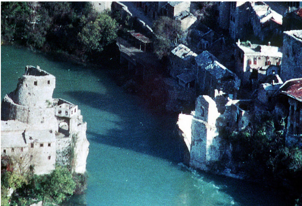
In November 1993, Croat armed forces shelled and destroyed Stari Most over the Neretva River, in Mostar, Bosnia and Herzegovina. © 1993 AP Photo/Zoran Bozicevic
